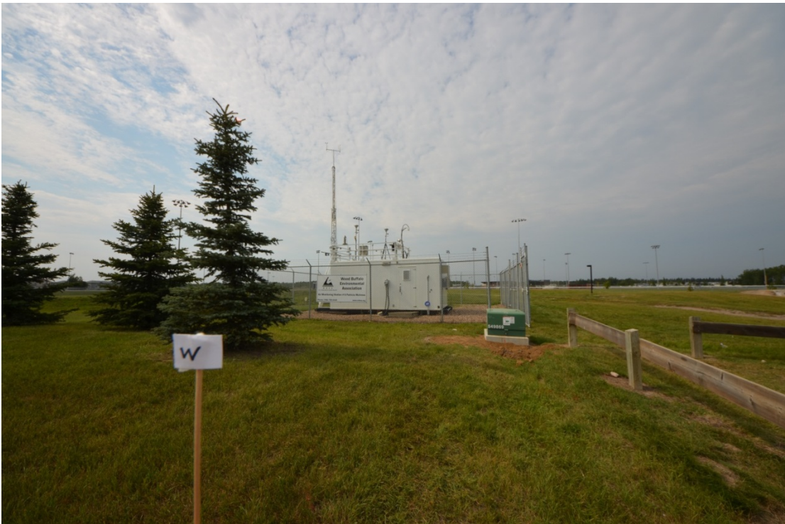
Figure 4.0 – Exterior of monitoring station looking west
