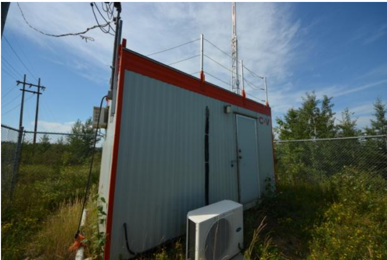
Figure 4.0 – Exterior of monitoring station
