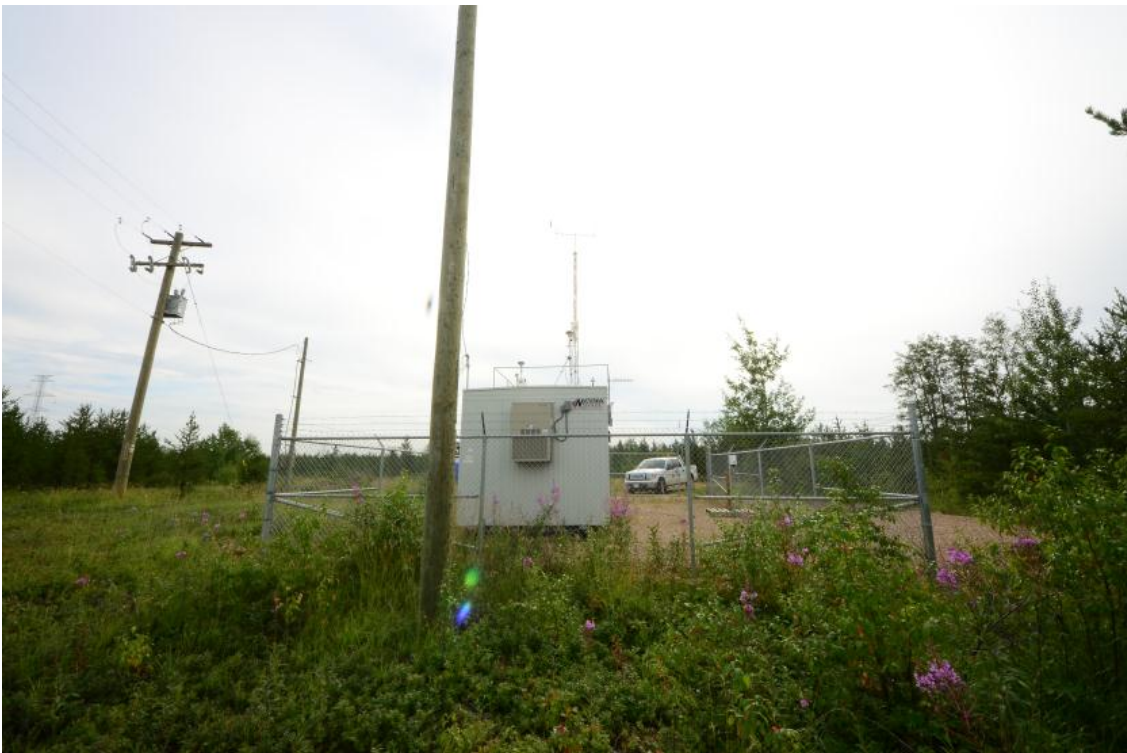
Figure 4.7 – Environ looking East
