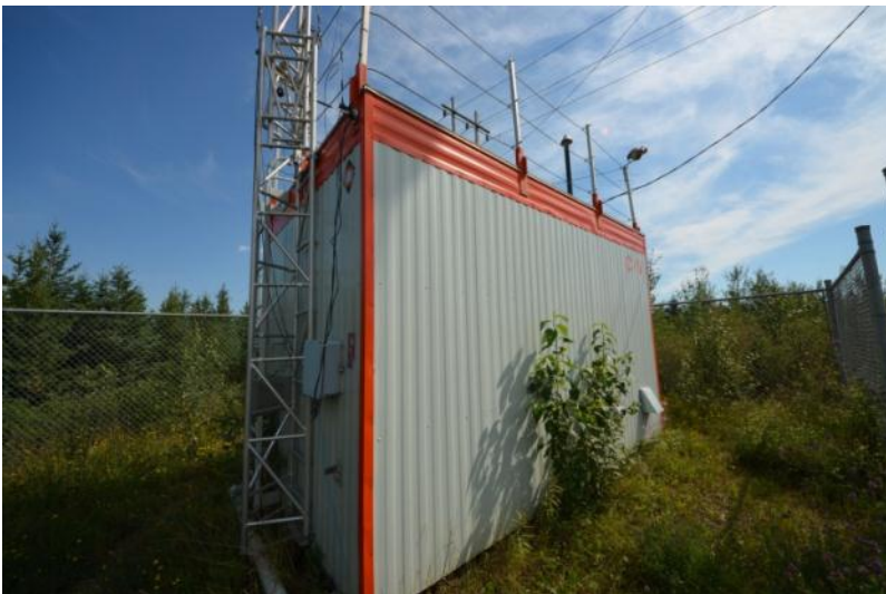
Figure 4.1 – monitoring compound looking south
