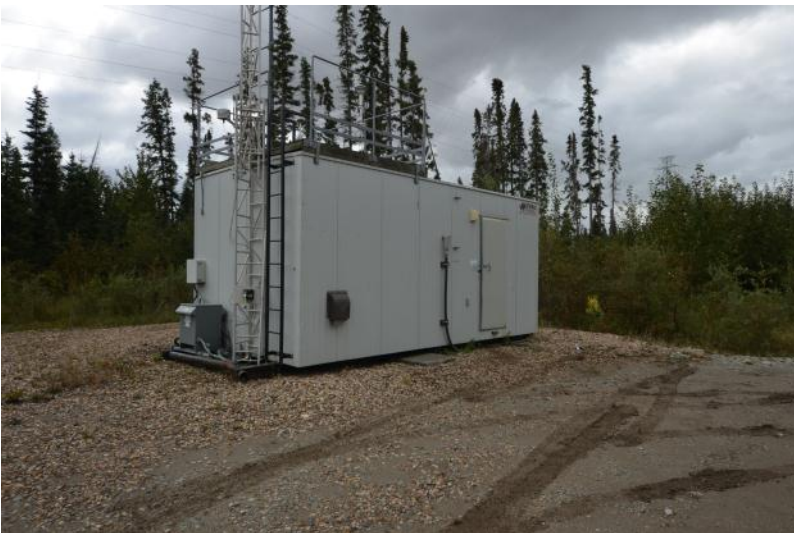
Figure 4.1 – monitoring compound looking south
