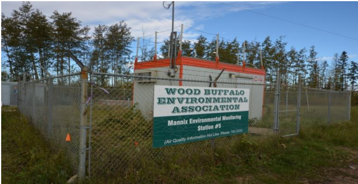
Figure 4.0 – Exterior of monitoring station
