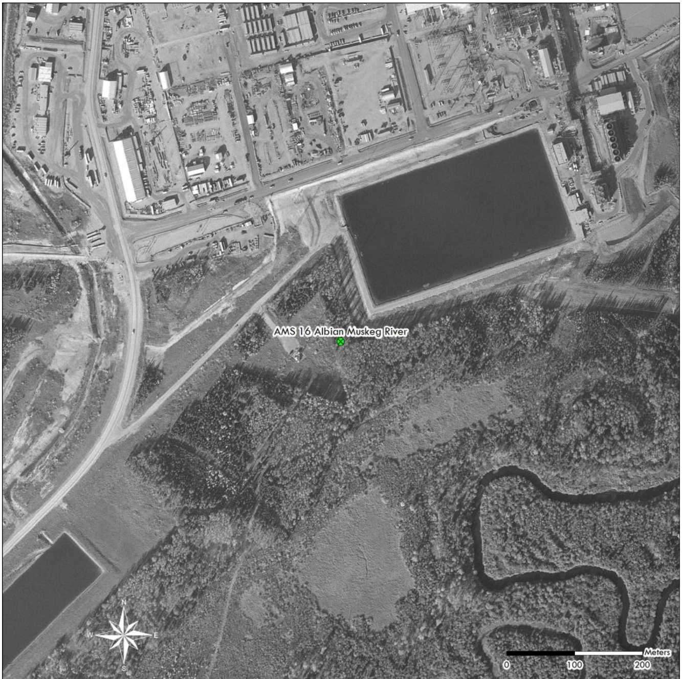
Figure 3.0 – Aerial photo showing AMS 16 – Shell Muskeg River Station
