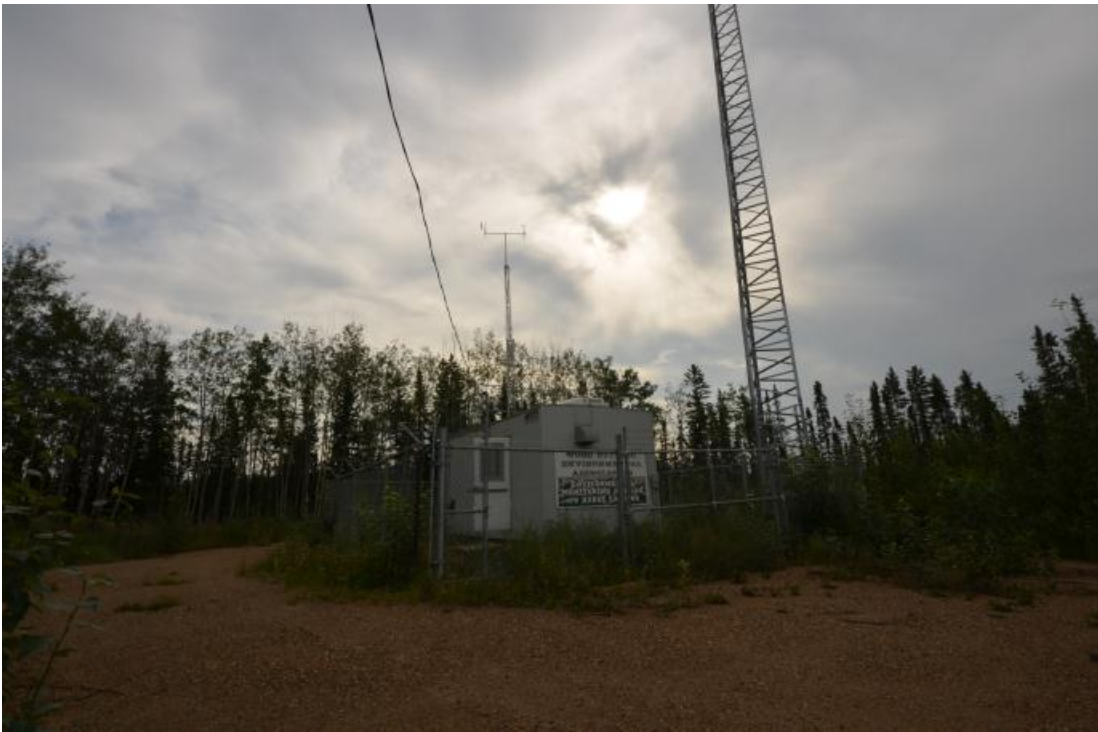
Figure 4.0 – Exterior of monitoring station
