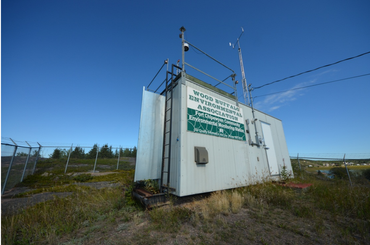
Figure 4.6 – Exterior of station looking North
