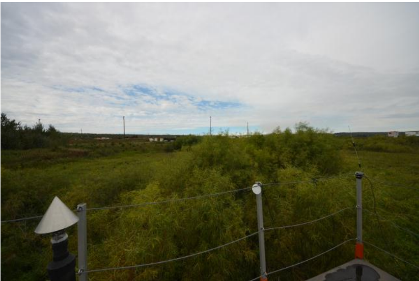
Figure 4.8 – Outdoor Sample Inlet & Indoor Sample Manifold
