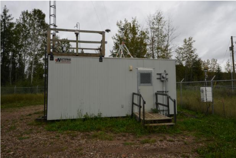
Figure 4.0 – Exterior of monitoring station
