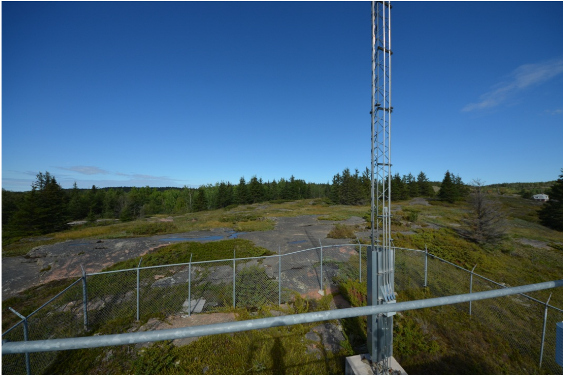
Figure 4.0 – Exterior of monitoring station looking North
