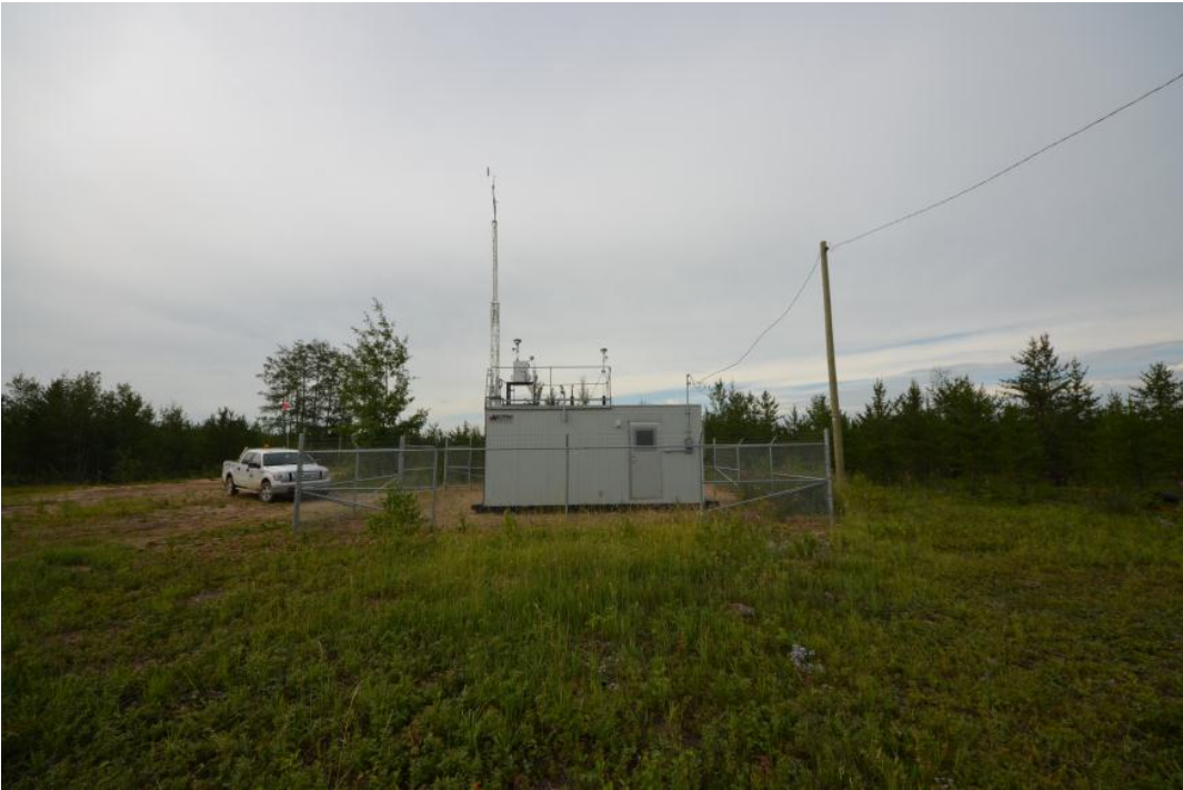
Figure 4.0 – Exterior of monitoring station
