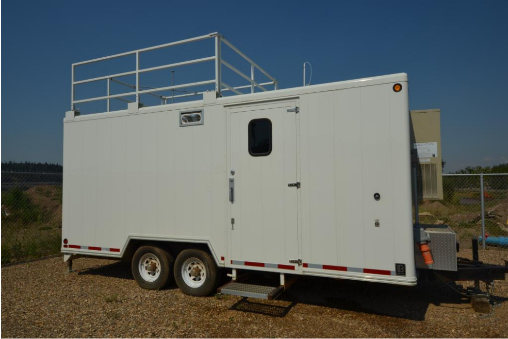
Figure 4.0 – Exterior of monitoring station
