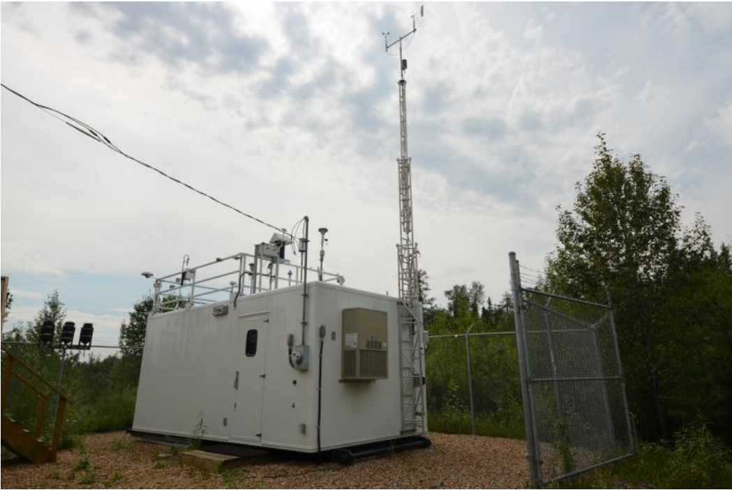
Figure 4.0 – Exterior of monitoring station
