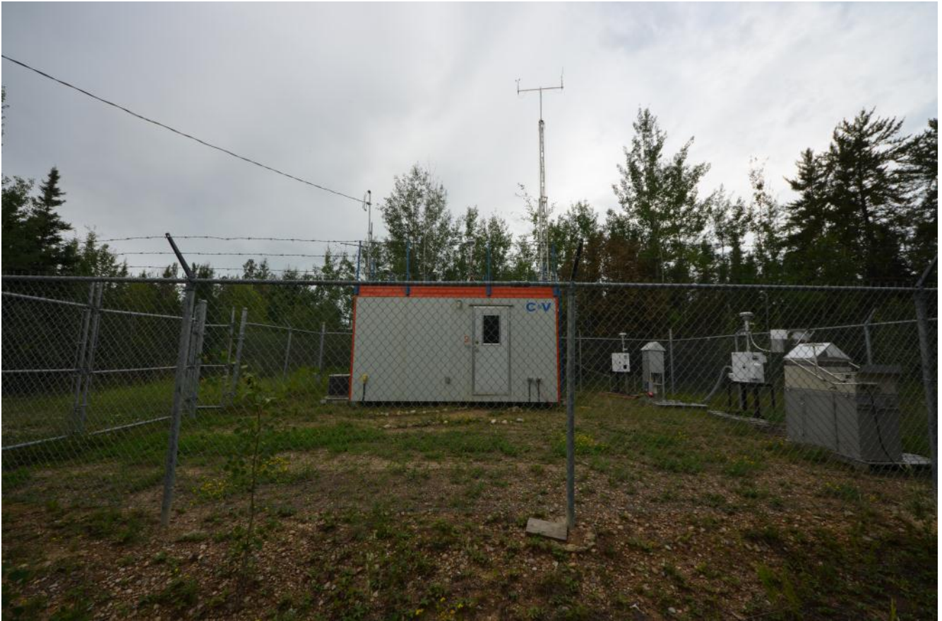
Figure 4.1 – Exterior of monitoring station
