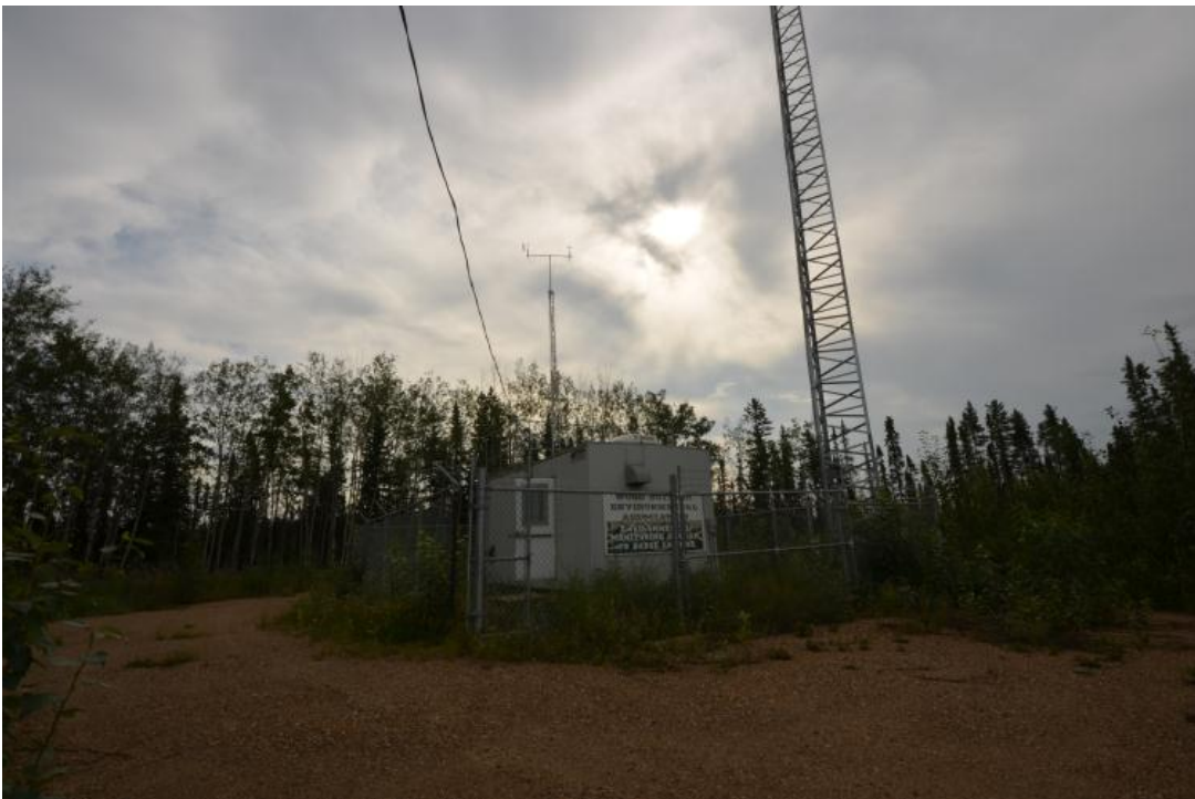
Figure 4.7 – Environ looking East
