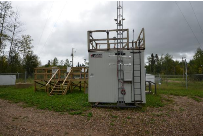
Figure 4.1 – monitoring compound looking south
