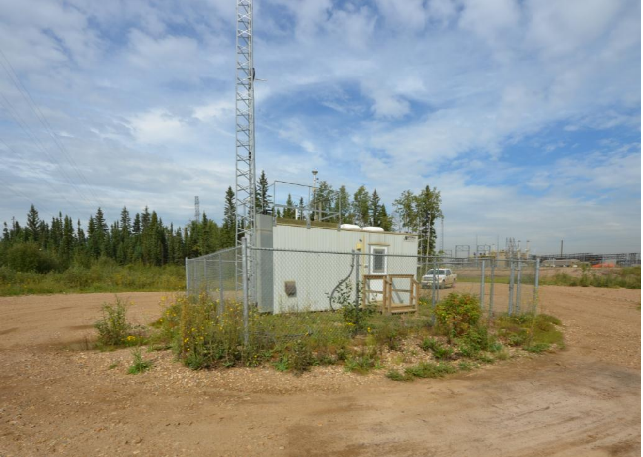
Figure 4.0 – Exterior of monitoring station looking North
