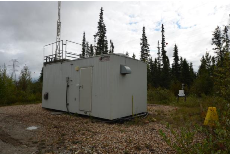
Figure 4.0 – Exterior of monitoring station
