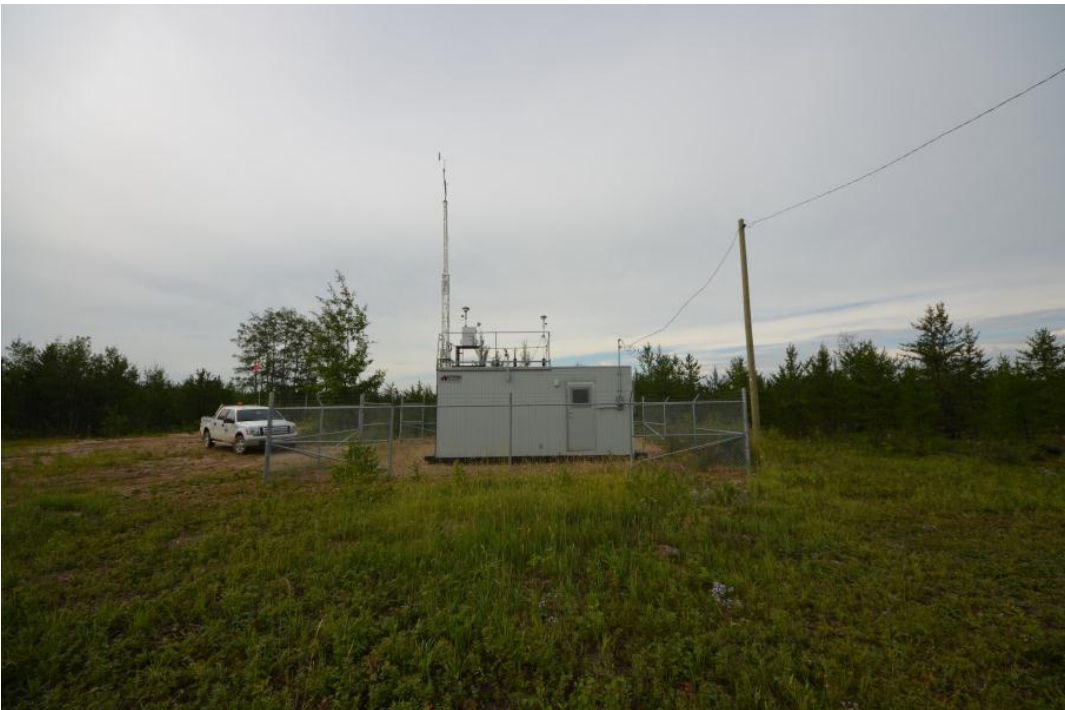
Figure 4.1 – monitoring compound looking south
