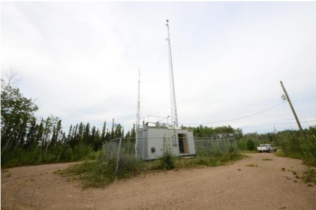
Figure 4.1 – monitoring compound looking south
