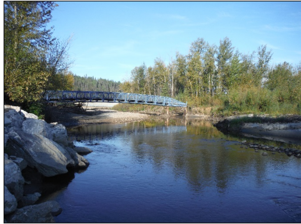
Water Quality Station HAR-1A: Right Downstream Bank, facing upstream
