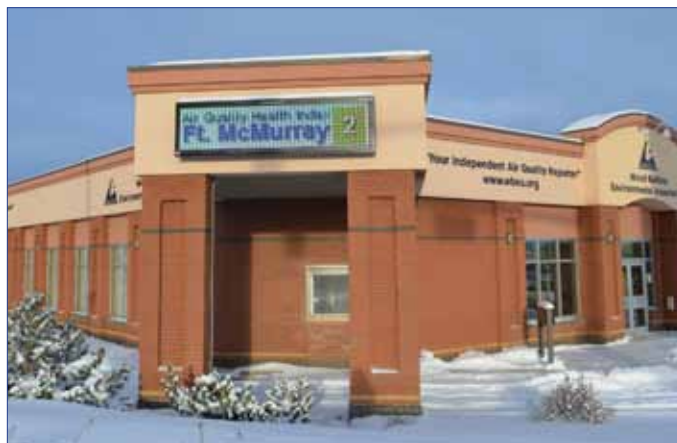
WBEA Headquarters with Electronic Message Centre.
